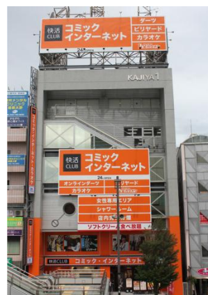
Sagamiono-ekimae Store (Kanagawa, Opened in July 2015)
